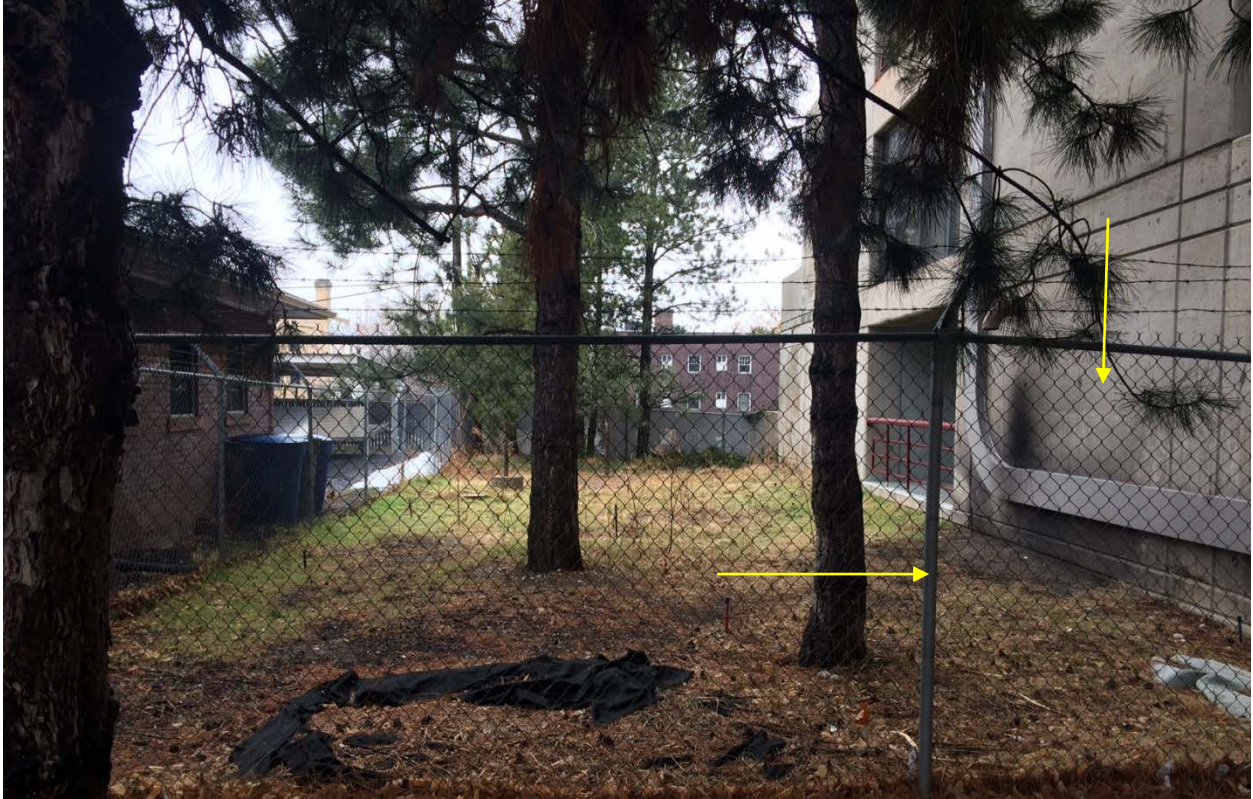
View from the east side of the subject property looking south. The proposed location of the electrical equipment is identified with yellow arrows. The accessory structure seen on the adjacent lot in the photo provides screening for the equipment.
